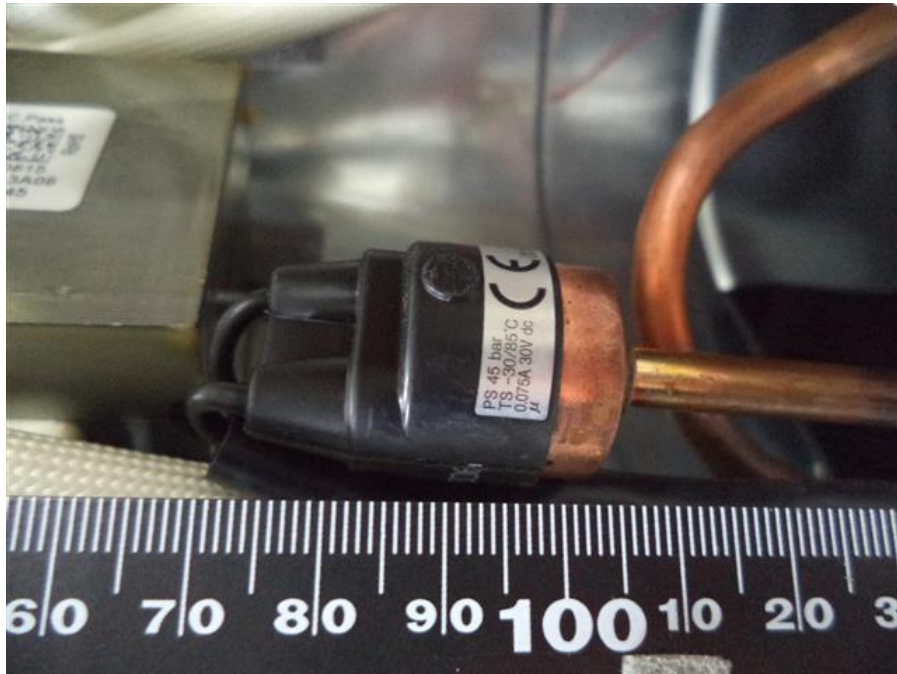
147. RAS-2M10U2AVG-E, High-Pressure Switch
