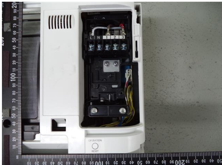
84. RAS-B16BKVGE, Terminal supply, interconnecting terminal and cord anchorage
