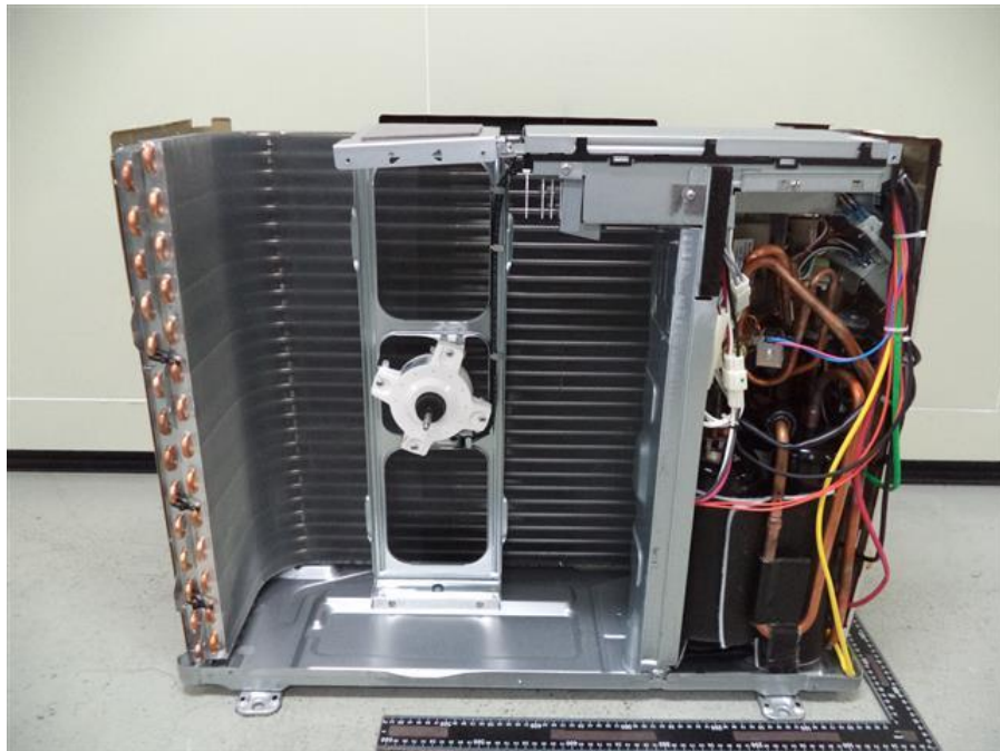
186. RAS-3M18U2AVG-E, Internal view removed fan blade
