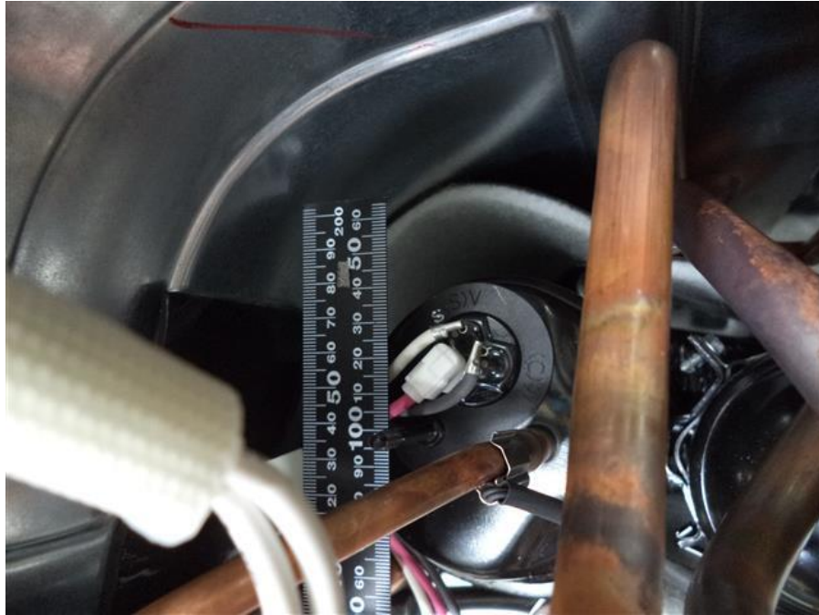
139. RAS-2M10U2AVG-E, Terminal of motor compressor
