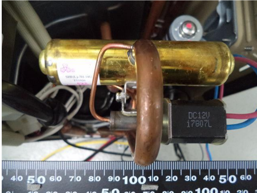
197. RAS-3M18U2AVG-E, 3 Way Valve Coil
