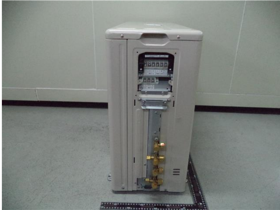
155. RAS-2M14U2AVG-E, Terminal block for supply main, interconnecting cable and cord anchorage
