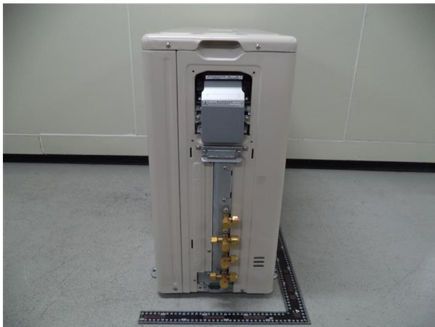
154. RAS-2M14U2AVG-E, Refrigerant connection
