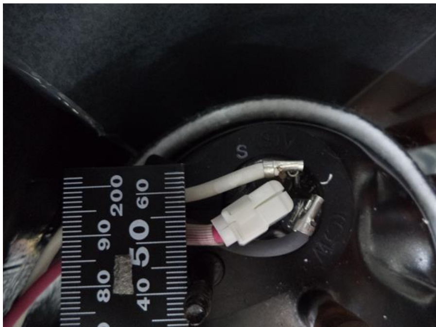
164. RAS-2M14U2AVG-E, Terminal of motor compressor
